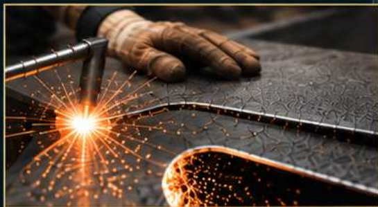
Fabrication of chainplate plates.
